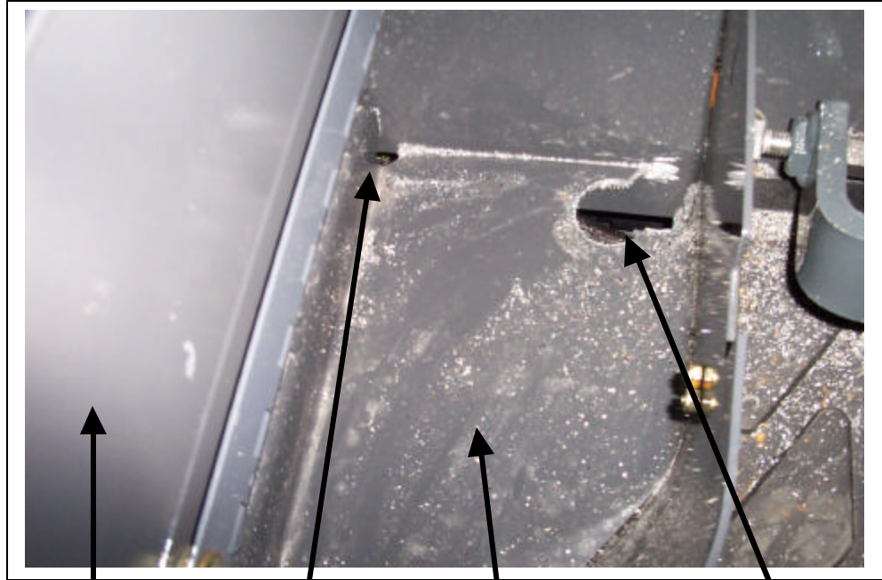
Run drain hose through this existing hole
